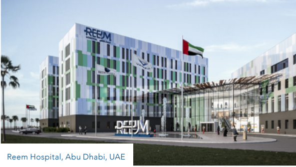
Reem Hospital, Abu Dhabi, UAE
